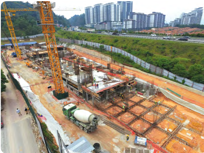
^ UEM Sunrise's affordable housing project Kiara Kasih undergoing construction
